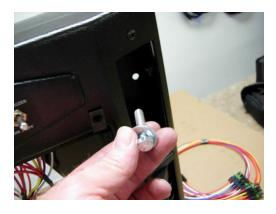
There are 4 holes (one in each corner) that will align with the unit, make sure the blower outlet is to the side of the switches of the console. Use 5/16 - 18 bolts with a flat washer (not provided), size accordingly to your roof thickness. You may need to seal the discharge area with foam to direct air into console
