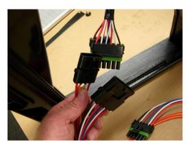
Clip the water tight connections together and push the wires back up into the return air side of the unit.
